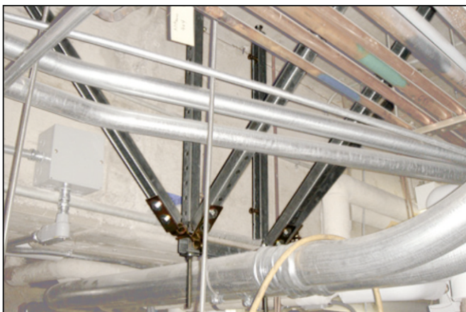
Figure 3.7, 3.8, 3.9, 3.10 Rigid Seismic Bracing (Steel Strut) Applications on Cable Trays and Conduits (Images from Federal Emergency Management Agency Website, www.fema.gov )
