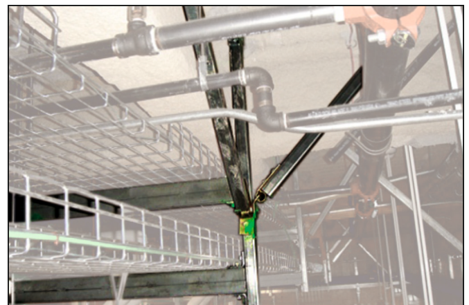
Figure 3.7, 3.8, 3.9, 3.10 Rigid Seismic Bracing (Steel Strut) Applications on Cable Trays and Conduits (Images from Federal Emergency Management Agency Website, www.fema.gov )
