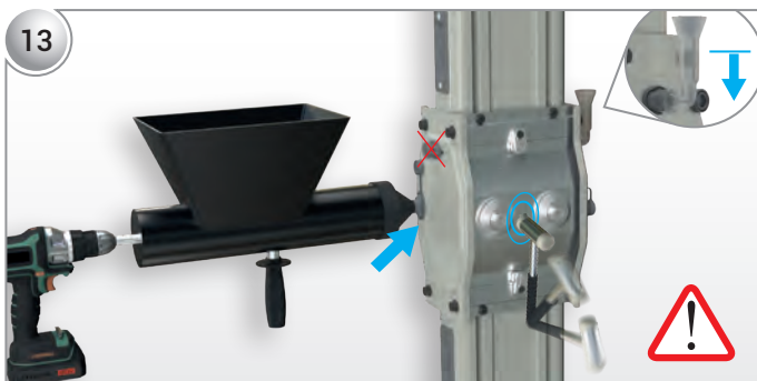
After the initial filling, tap the busbar block joint from underneath with a plastic mallet. If a drop in the Flex-Comp level is observed in the level control plastic, continue the filling process.
